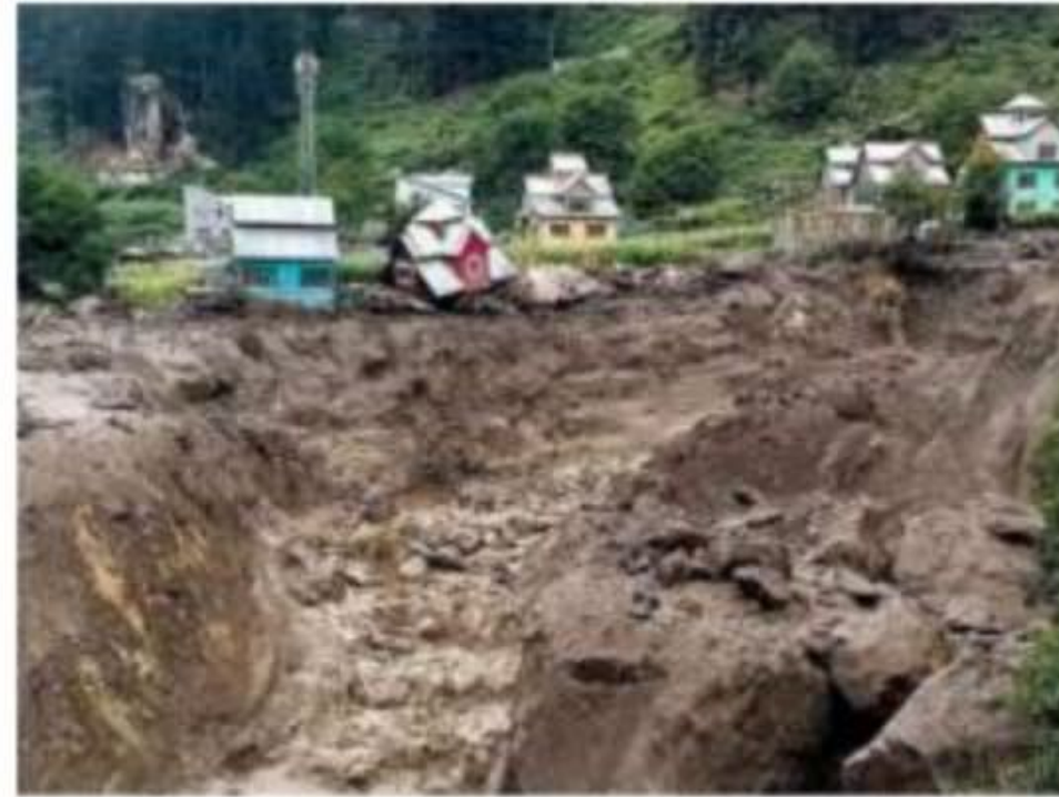
Washed away: An area damaged in the flash flood in Kishtwar district of Jammu and Kashmir on Thursday. PTI
